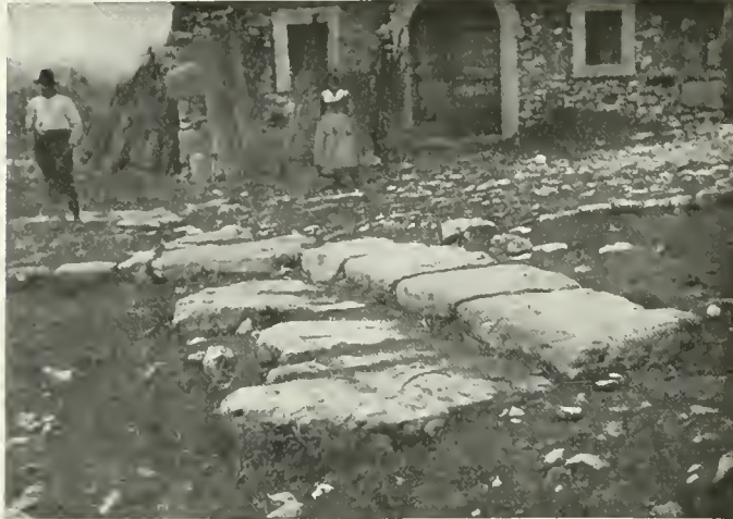
FIGURE 7. — ANCIENT ROAD-PAVEMENT AT THE THIRD FORK, 17
